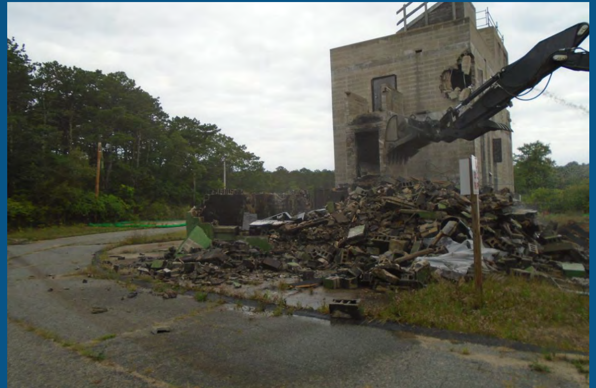
August 2021: Burn Building Demolition
