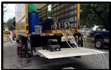
Chemical Oxidation & Surfactant Injections
