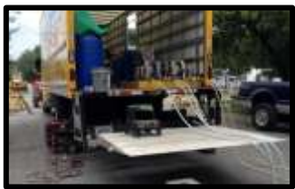
Chemical Oxidation & Surfactant Injections
