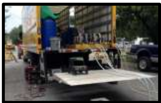
Chemical Oxidation & Surfactant Injections
