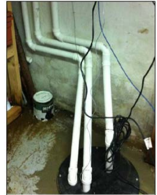
Covered sump with vent and discharge pipes (from VT VI Guidance)
