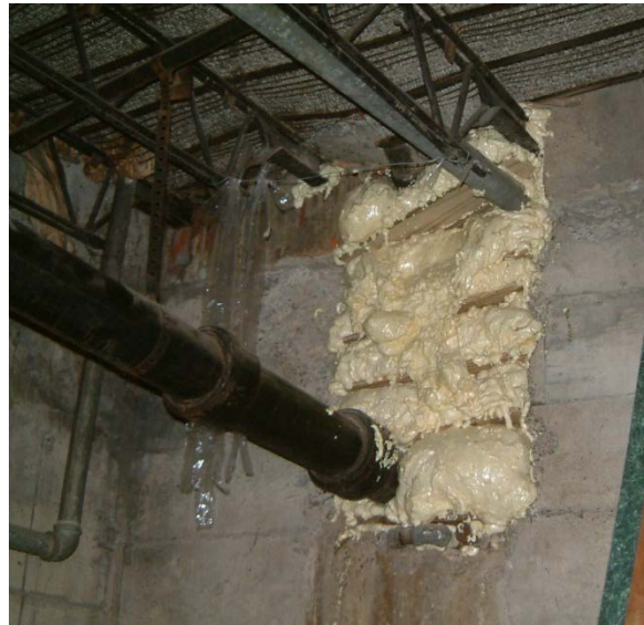
Utility penetration sealed with spray foam
