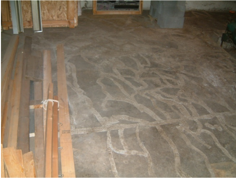
Floor cracks/joints sealed with sealant or caulk
