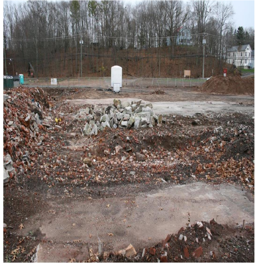
9. General view of the existing foundation and rubble, looking easterly;
