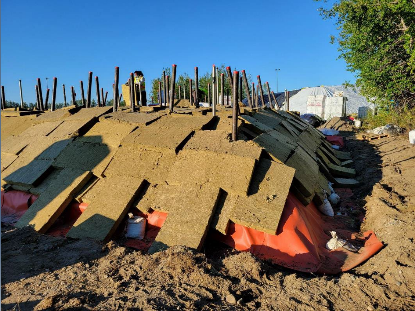
Stockpile covered with impermeable barrier & insulating mineral wool
