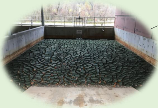
Waterbury, sludge drying beds
