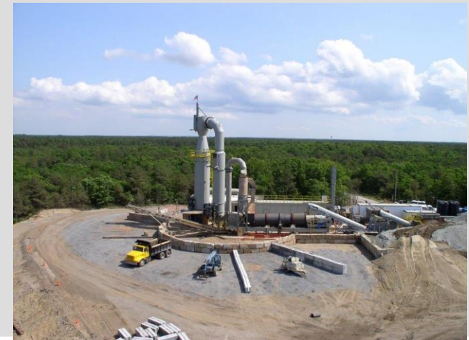
Typical Layout of a Thermal Desorption Project
