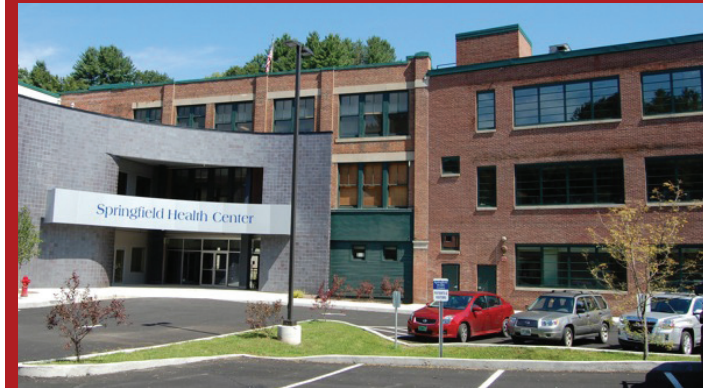
Gear Shaper Facility – before and after
