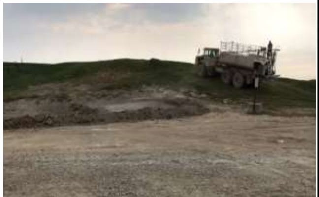
SPRAYING ALTERNATE DAILY COVER
