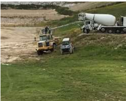
LOADING SPRAYER TRUCK
