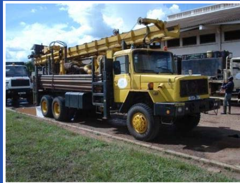
Materials to Site
