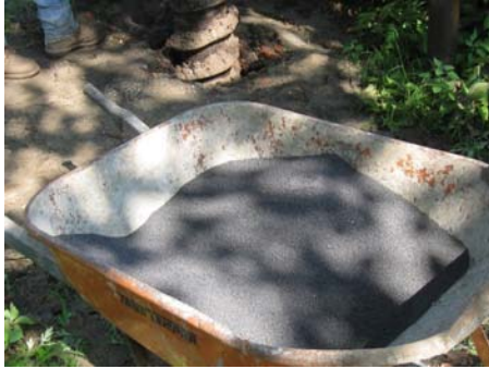
Above: Conductive Backfill Material (Graphite) Right: Electrode before connections and capping
