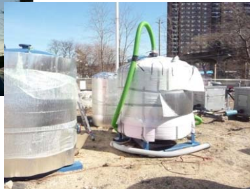
Insulated GAC Vessels (2x 5,000 lb vessels and 2x 2,000 lb vessels)
