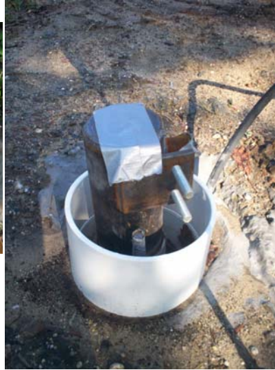
Above: Conductive Backfill Material (Graphite) Right: Electrode before connections and capping
