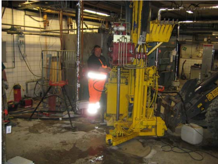
Drilling between dry cleaning machines, walls, cables and pipes
