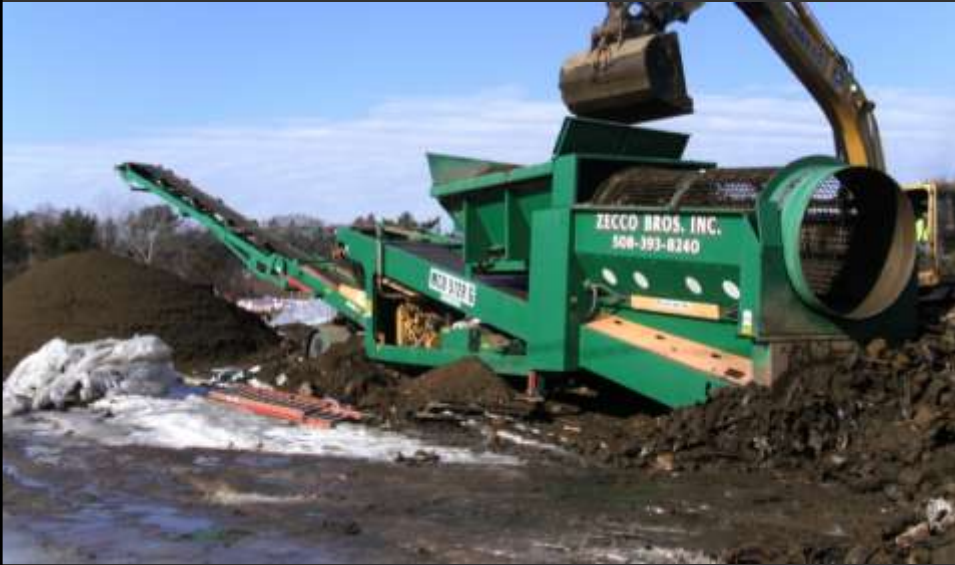
Trommel screen for physical separation of debris from soil
