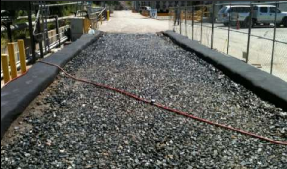
Decontamination pad for trucks and excavators (CA)
