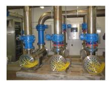
The photograph to the left is of ultraviolet (UV) germicidal lamps which are used for water disinfection/sanitation at one Massachusetts drinking water treatment facility. There are three UV disinfection systems, each with approximately 40 lamps. Each UV lamp contains less than 5 milligrams to more than 1,000 milligrams (1 gram) of mercury.
