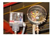
The photograph to the left shows a Pressuretrol<sup>TM</sup> (left) and a pressure gauge that contains a mercury switch (right) used at a Massachusetts wastewater treatment facility. The facility also uses non-mercury pressure gauges as shown in the two photographs described below.
