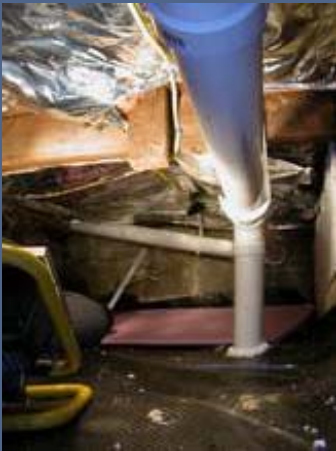
View of a newly installed vapor barrier membrane and SSD suction piping
