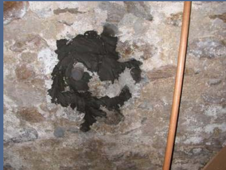
View of a sealed piping penetration
