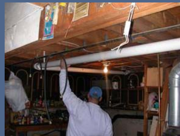
Placement of SSD piping into the ceiling rafters
