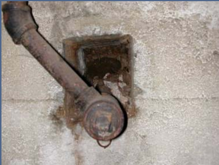
View of a piping penetration in need of sealing
