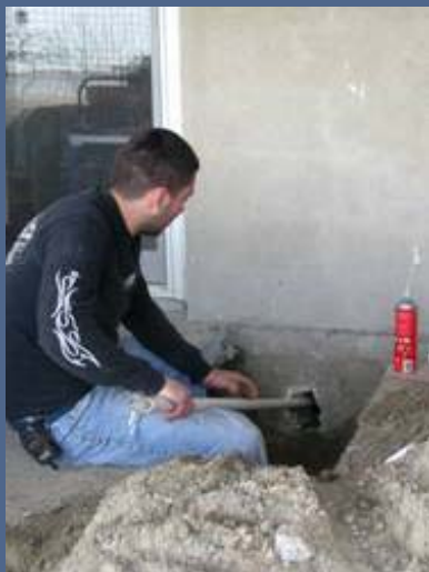
Excavation of a horizontal suction hole
