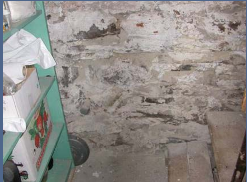
Crumbling high lime mortar in the fieldstone walls
