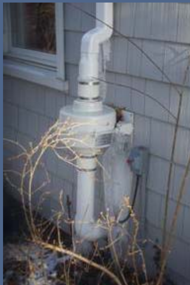
Views of icing build-up on SSD fans
