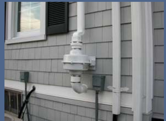
View of exterior SSD system components; a GP501 fan, on/off switch, downspout, and exhaust vent cap
