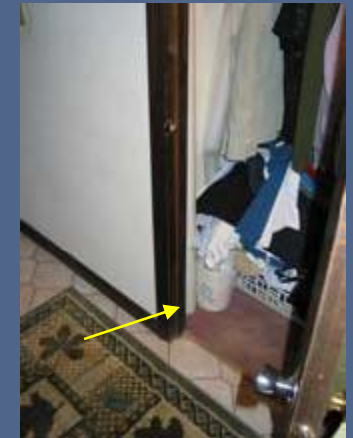
View of hidden SSD piping in a closet
