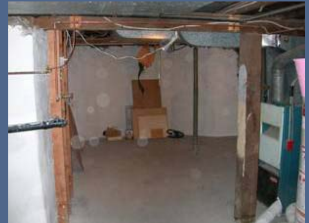
Newly installed concrete slab (also visible are the newly parged walls)
