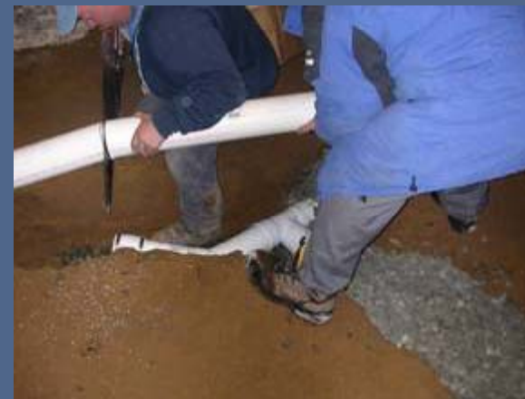
Placement of underground SSD piping prior to pouring a new basement slab
