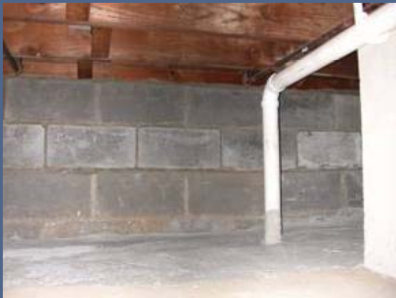
View of a newly poured concrete crawlspace slab and SSD suction piping
