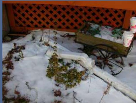
Views of broken exhaust piping
