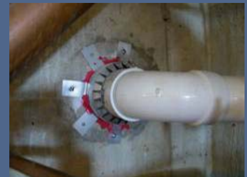
View of a Fire Collar installed to maintain fire code at the apartment buildings
