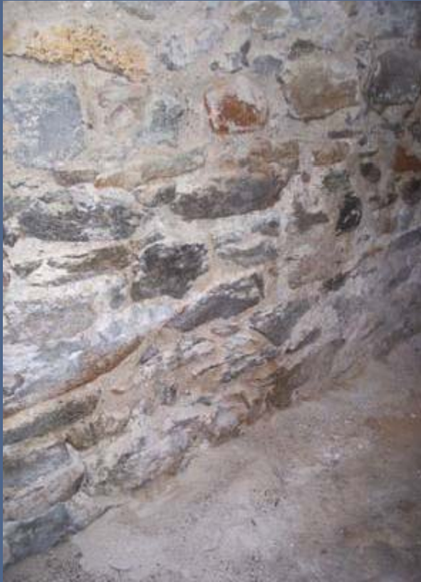
Crumbling high lime mortar fieldstone walls before parge coat
