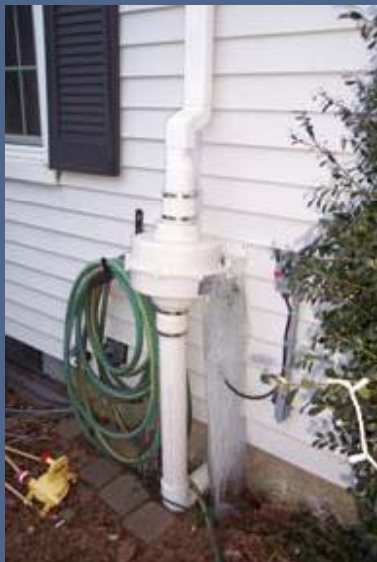
Views of icing build-up on SSD fans
