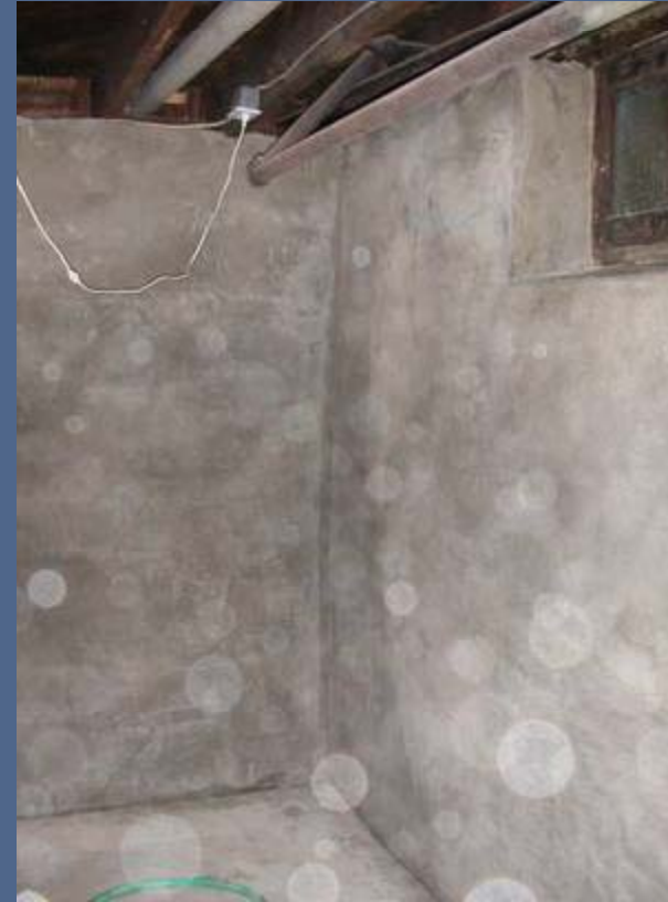
View of the fieldstone walls after a parge coat has been applied
