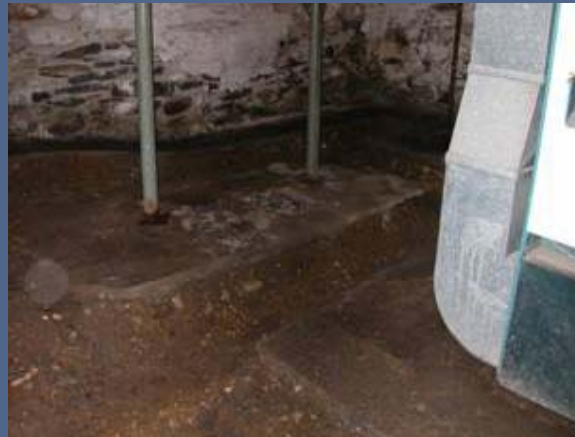
Concrete slab, during demolition (also visible are the fieldstone walls)
