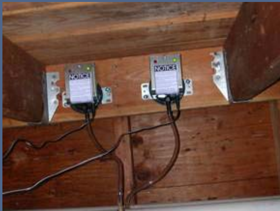
View of two SSD monitoring systems
