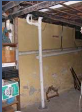
View suction piping (both for the main slab and a crawlspace)
