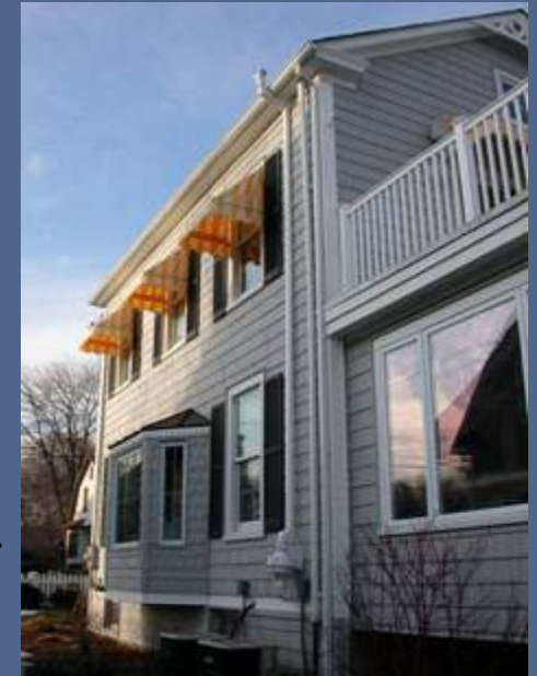
View of exterior SSD system components; a GP501 fan, on/off switch, downspout, and exhaust vent cap
