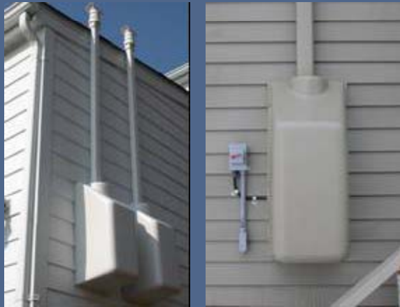
Views of exterior SSD system components; covered GP501 fans, on/off switches, downspouts, and exhaust vent caps
