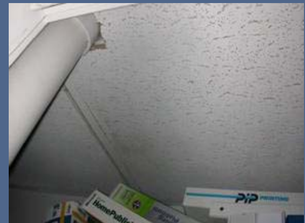
View of hidden SSD piping in a closet (in the drop ceiling)
