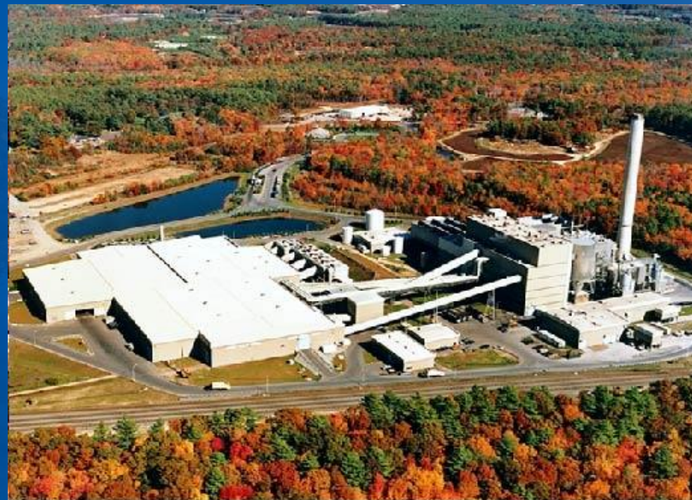
SEMASS RDF – 3,000 TPD
