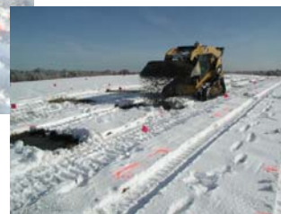
Gravel for Leveling
