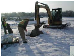
Removal of Vegetation
