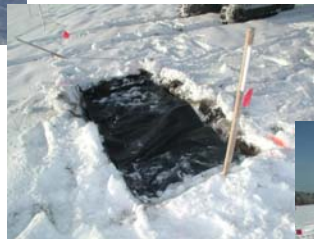
Placement of Geotextile
