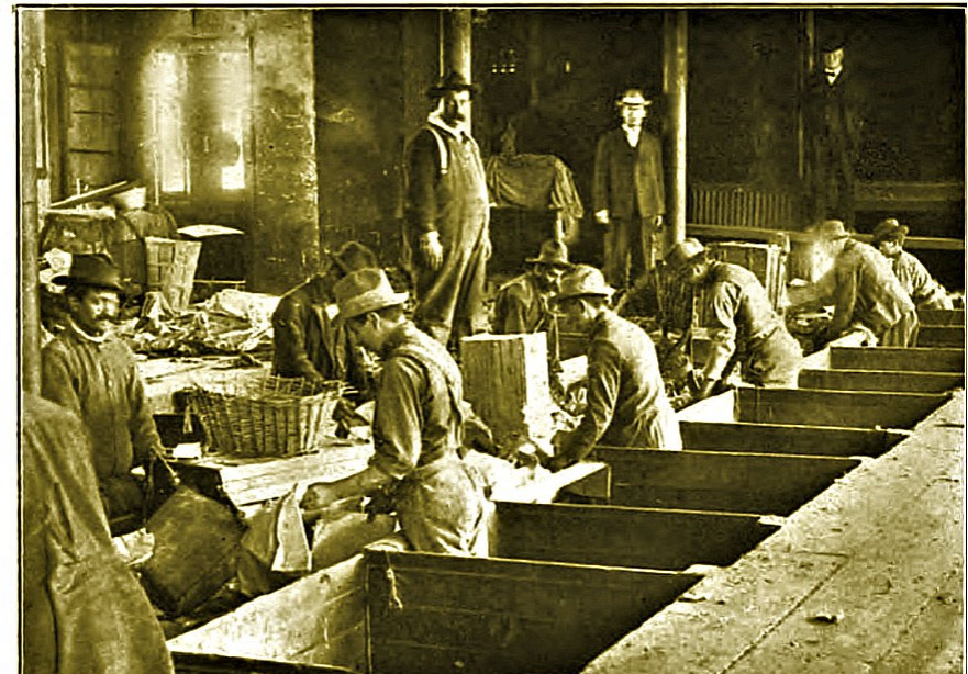
Sorting Refuse from Belt Conveyor at West 47 th NYC (1907) Photo by George Lane
