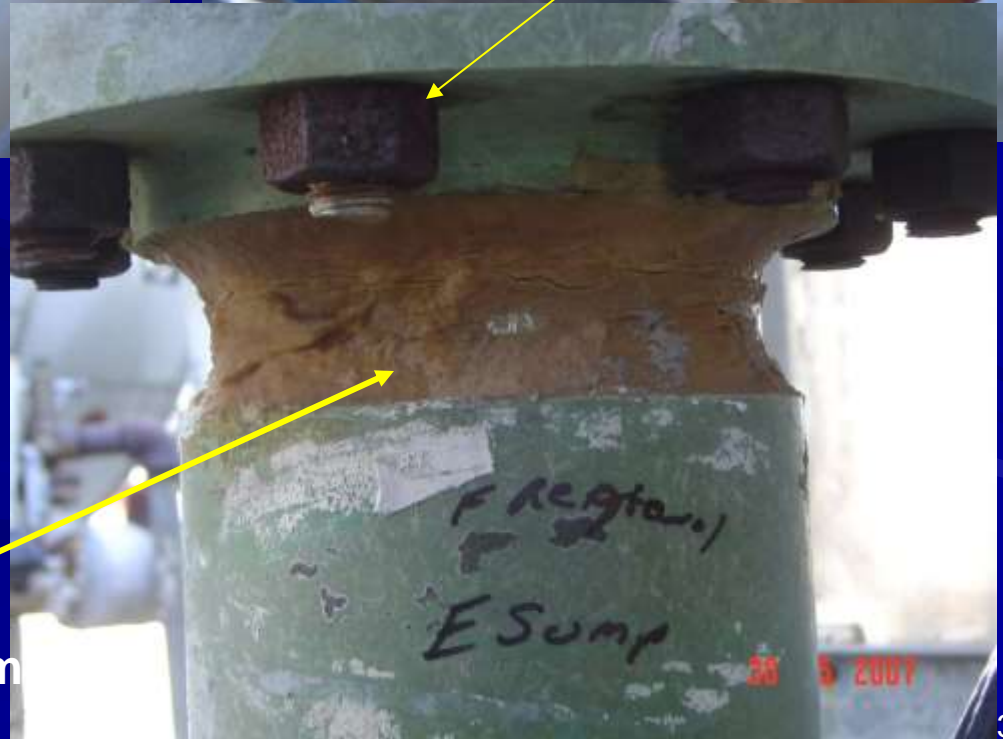
Flanges Missing Bolts & Washers
