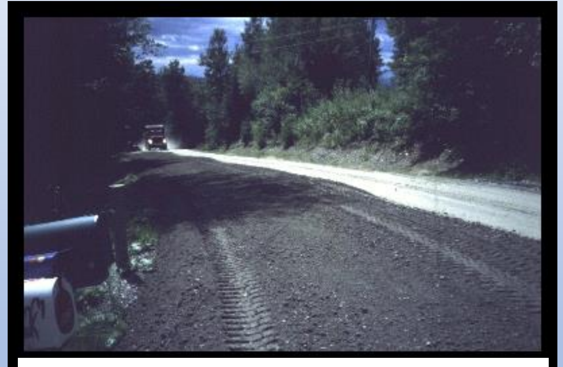
RAS/RAP/Gravel placement, Huntington, VT
