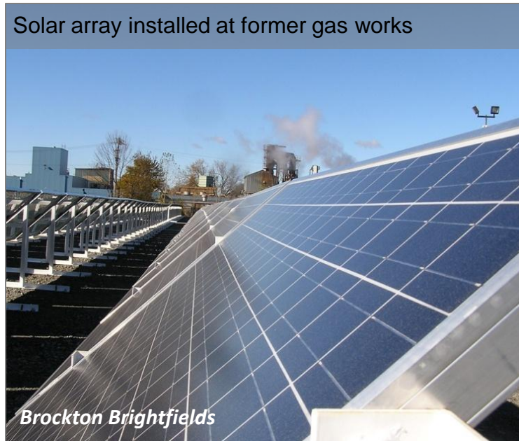
Fixed tilt system at landfill
