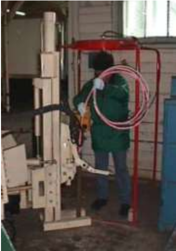
NAPL FLUTe Deployed in Direct Push Casing
