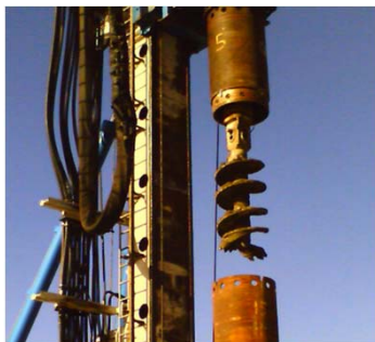
Large Diameter Boring Installation
