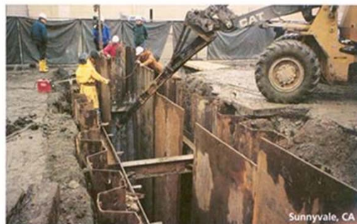
Conventional Excavate and Fill Installation with Sheet Piles
