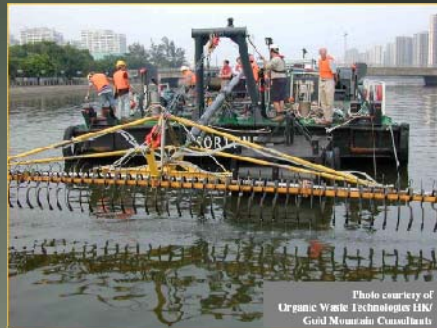
Limnofix In Situ Sediment Treatment Technology (LIST) (Golder Associates)
