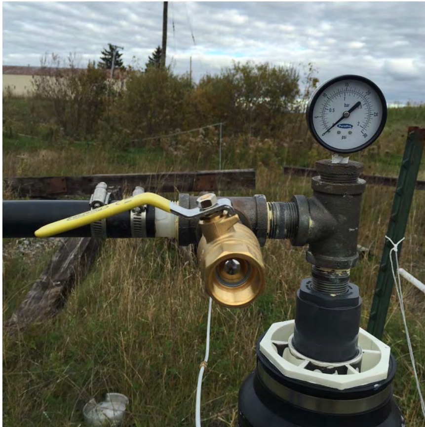
Relieve valve and well head assembly
