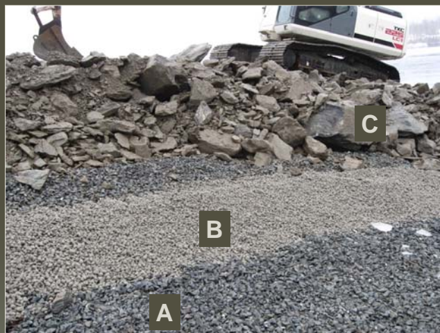
Placing Gas Transmission (A) & Control Layers (B), Armor (C) in Intertidal Zone Slide content courtesy of RMT, Inc
