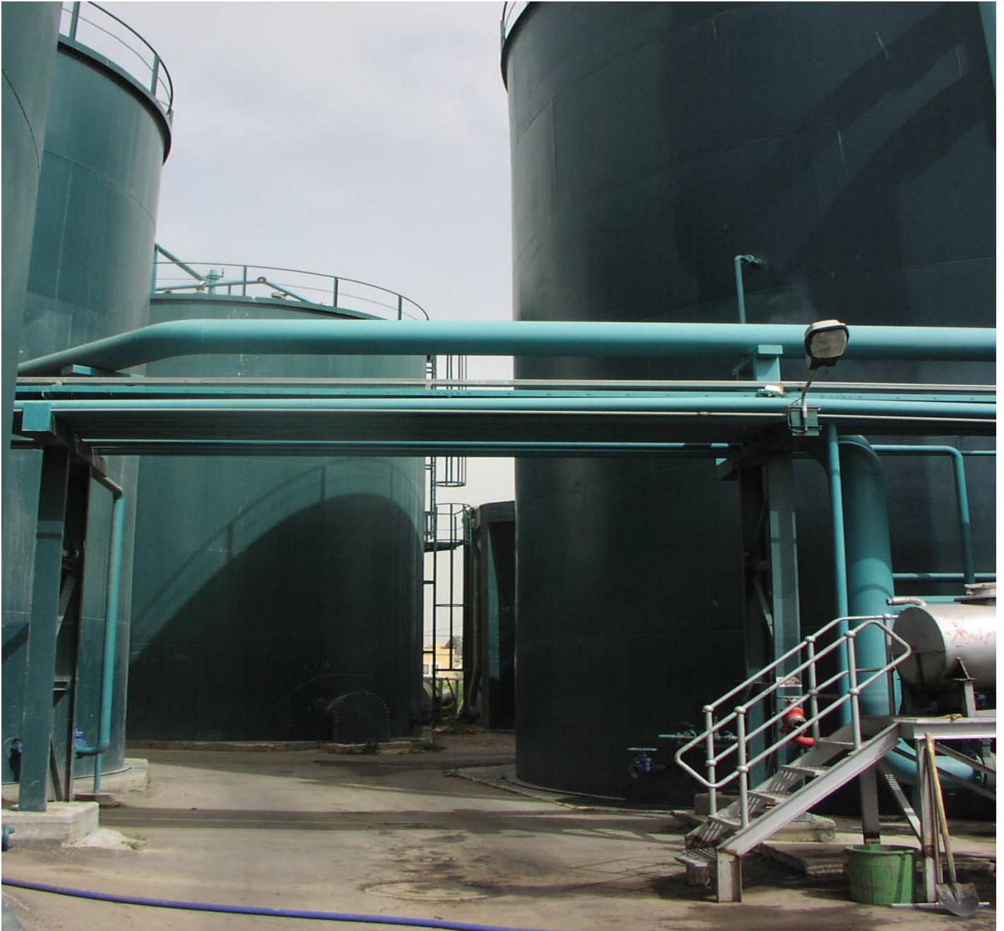
Digestion Tanks ArrowBio, Tel Aviv
