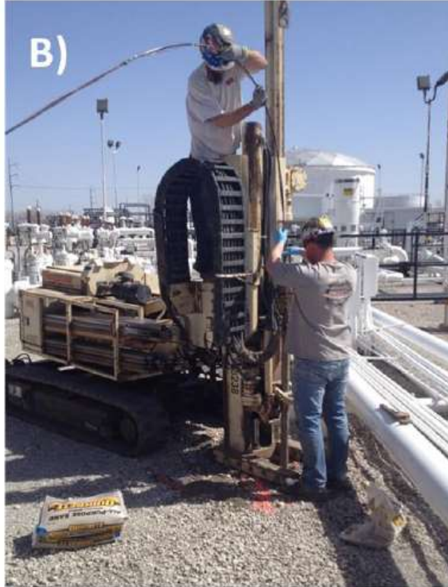
Installation of stick using direct push rig.
