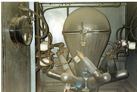
Mercury Arc Rectifier; Photo Source: Wikipedia
