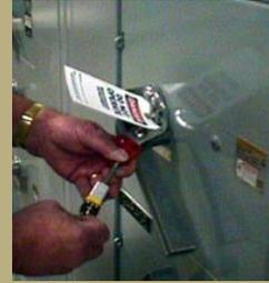
In a **tagout**, the energy-isolating device is placed in the "safe" position and a written warning is attached to it.
