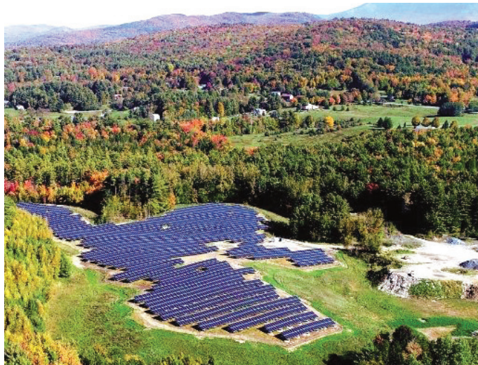
Solar Panels on a Closed Landfill
