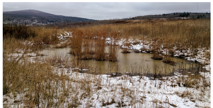
Ponding On a Landfill Due to Settlement
