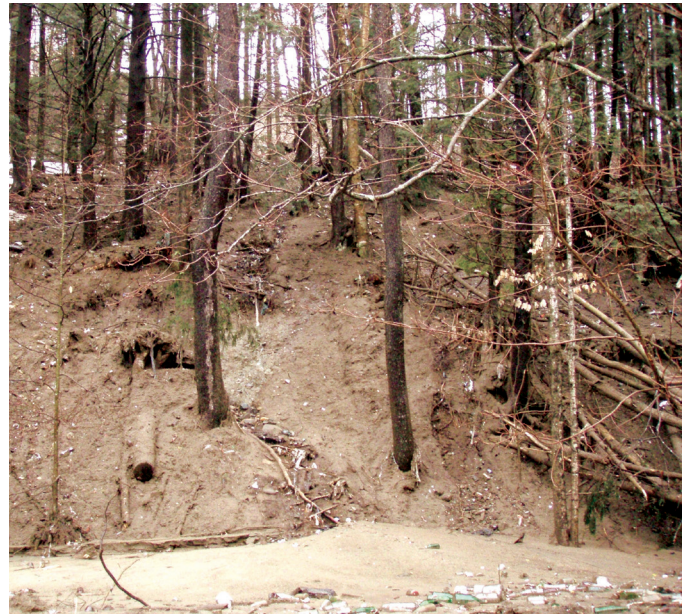
Old Landfill with Tree Growth and Erosion (note exposed waste in channels and at base)
