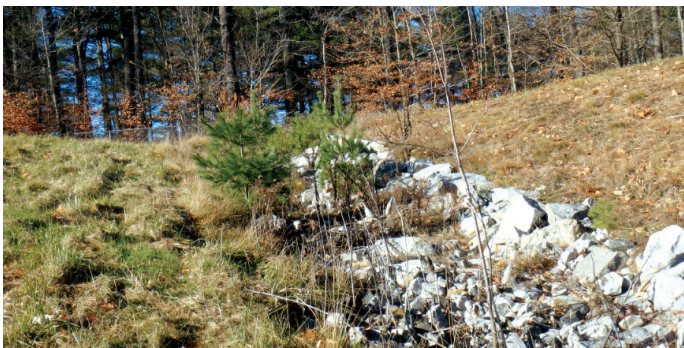
Woody Growth and Blocked Drainage Swale
