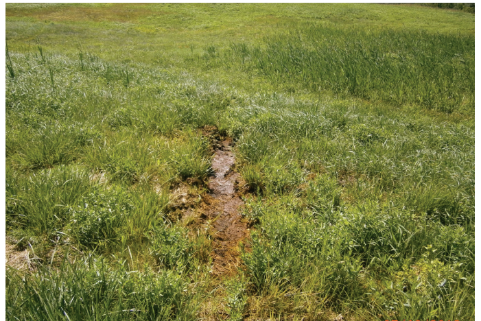
Leachate Seep on Landfill Side Slope
