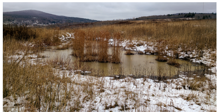
Ponding On a Landfill Due to Settlement
