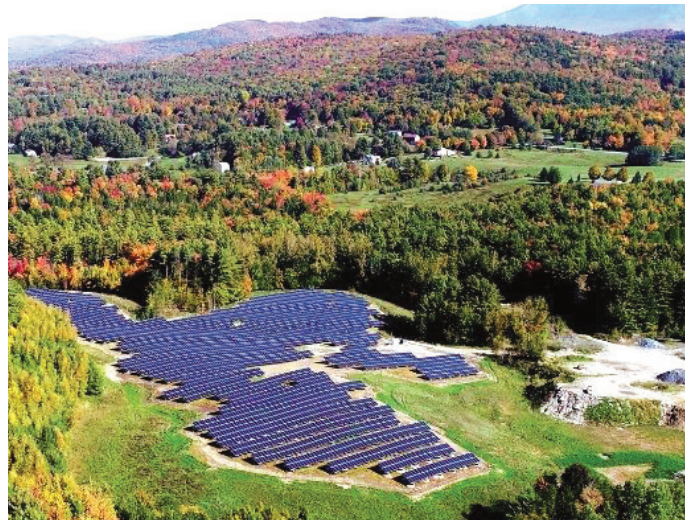
Solar Panels on a Closed Landfill
