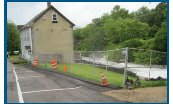
Mica Building, Bristol, NH – before, during, and after demolition
