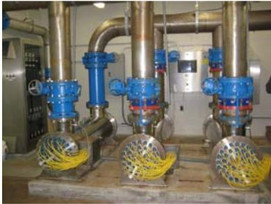
The photograph to the left is of ultraviolet (UV) germicidal lamps which are used for water disinfection/sanitation at one Massachusetts drinking water treatment facility. There are three UV disinfection systems, each with approximately 40 lamps. Each UV lamp contains less than 5 milligrams to more than 1,000 milligrams (1 gram) of mercury.
