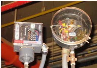
The photograph to the left shows a Pressuretrol™ (left) and a pressure gauge that contains a mercury switch (right) used at a Massachusetts wastewater treatment facility. The facility also uses non-mercury pressure gauges as shown in the two photographs described below.
