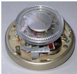
Mercury Switch inside Thermostat
