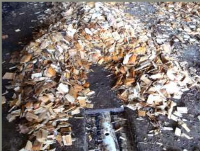
Woodchips over Cover Plates at the UNH Facility
