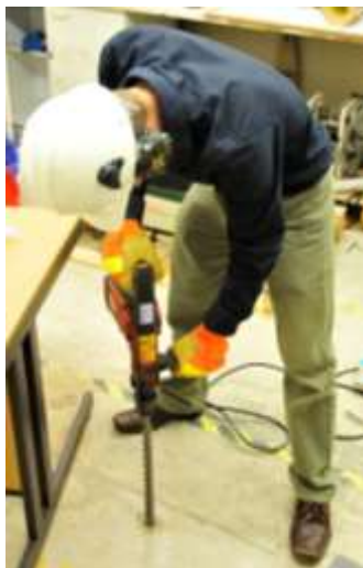
Temporary hole drilled through slab and sealed with hot beeswax
