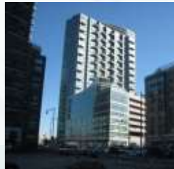
Northern edge of site boundary ~ 100 ft from high-rise, luxury residential building
