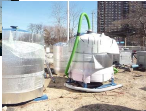
Insulated GAC Vessels (2x 5,000 lb vessels and 2x 2,000 lb vessels)
